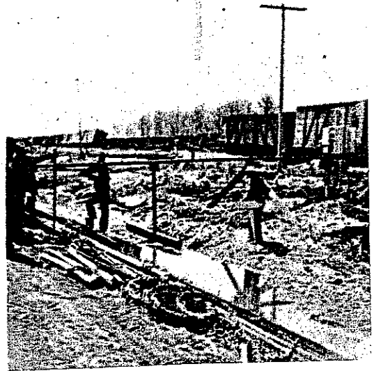
Cleanup and repair after Hickman flood of 1950
