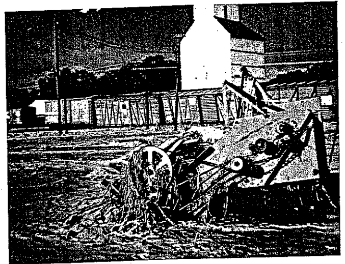
Damage from flood of 1950's
